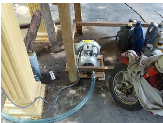
Air blowers create more oxygen for the biocatalysts to digest waste
