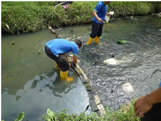
Retention treatment area allows more time for the biocatalysts to break down pollutants
